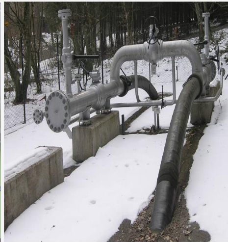
A pig launcher/receiver in Switzerland. Image: Wikimedia commons
